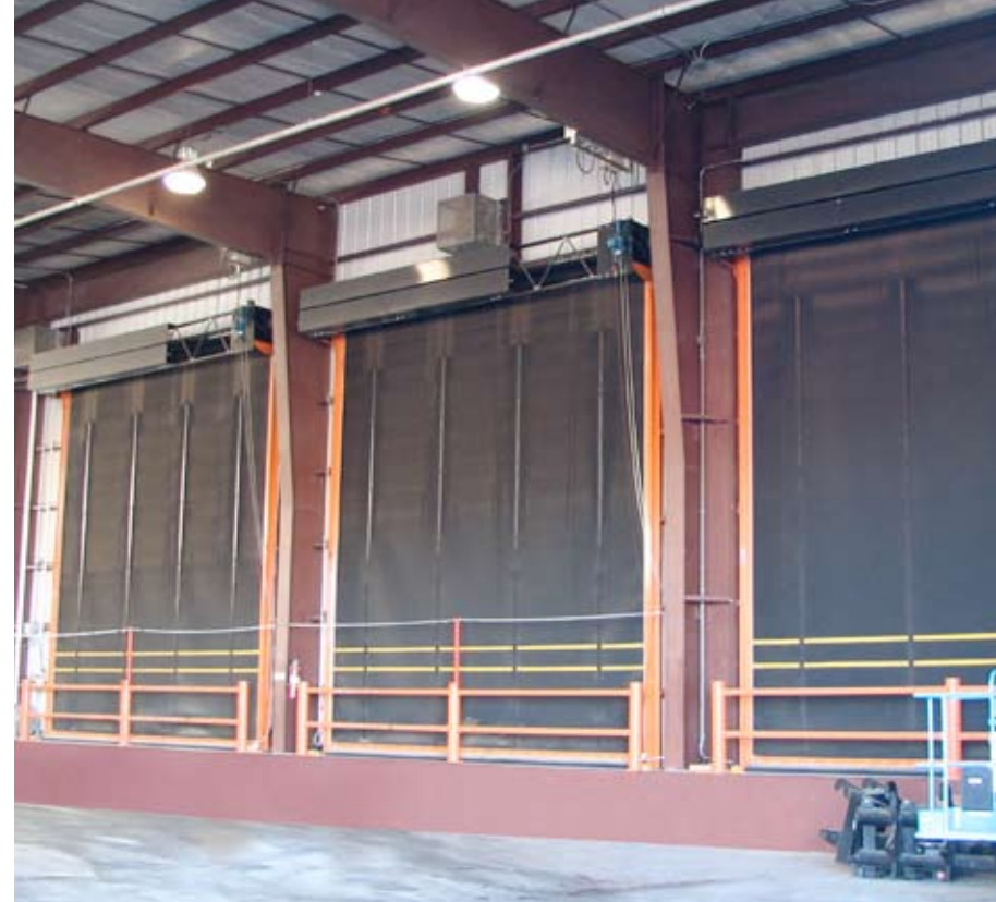
Waste Water Management
